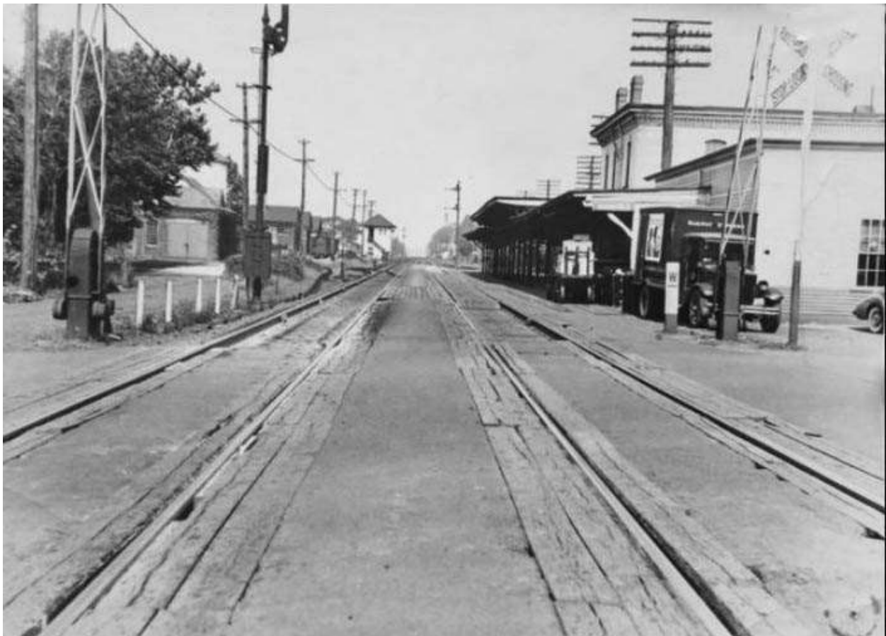
Above is the Chauncy Street grade crossing with arms designated to stop vehicular traffic.
