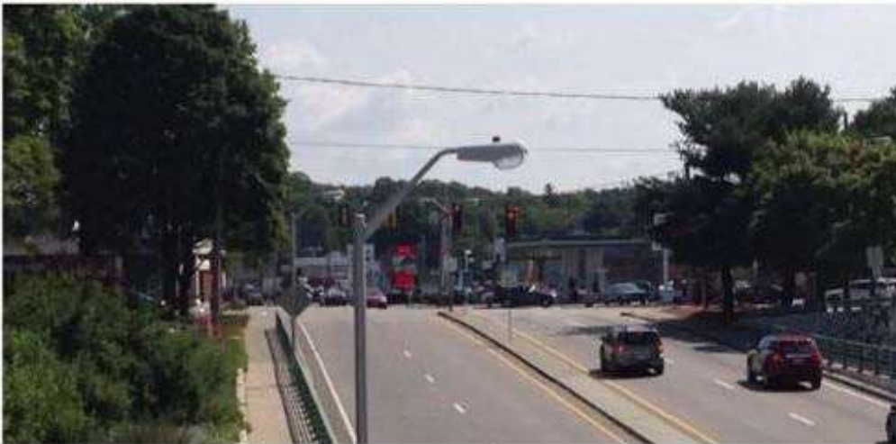
Above before and after views of the North Common and the Rt. 106 intersection with North Main Street. The area was transformed by the underpass project which eliminated grade-level train crossings.
