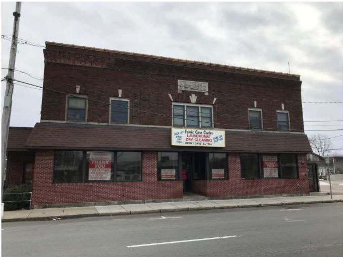
The Billings Building, once widely known as the A&P grocery store, dates to the early 1900s. In the 1970s the location was a Cumberland Farms store, and later became the Fabric Care Center. [Courtesy/Mansfield Historical Society]
