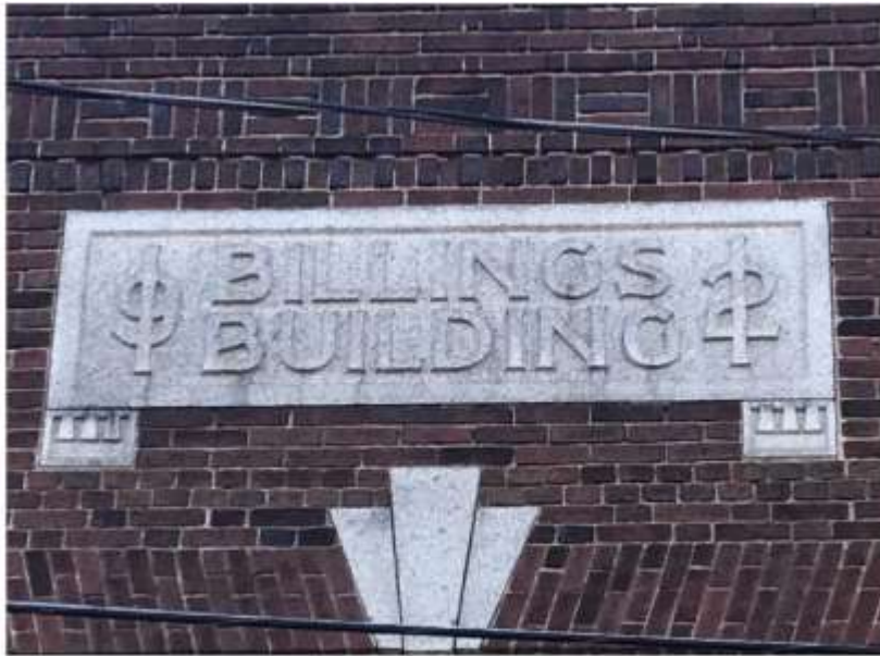
Also slated to come down is the Billings Building of Thomas Street, once widely known as the A&P grocery store, and better known in recent years as the Fabric Care Center. [Courtesy/Mansfield Historical Society]
