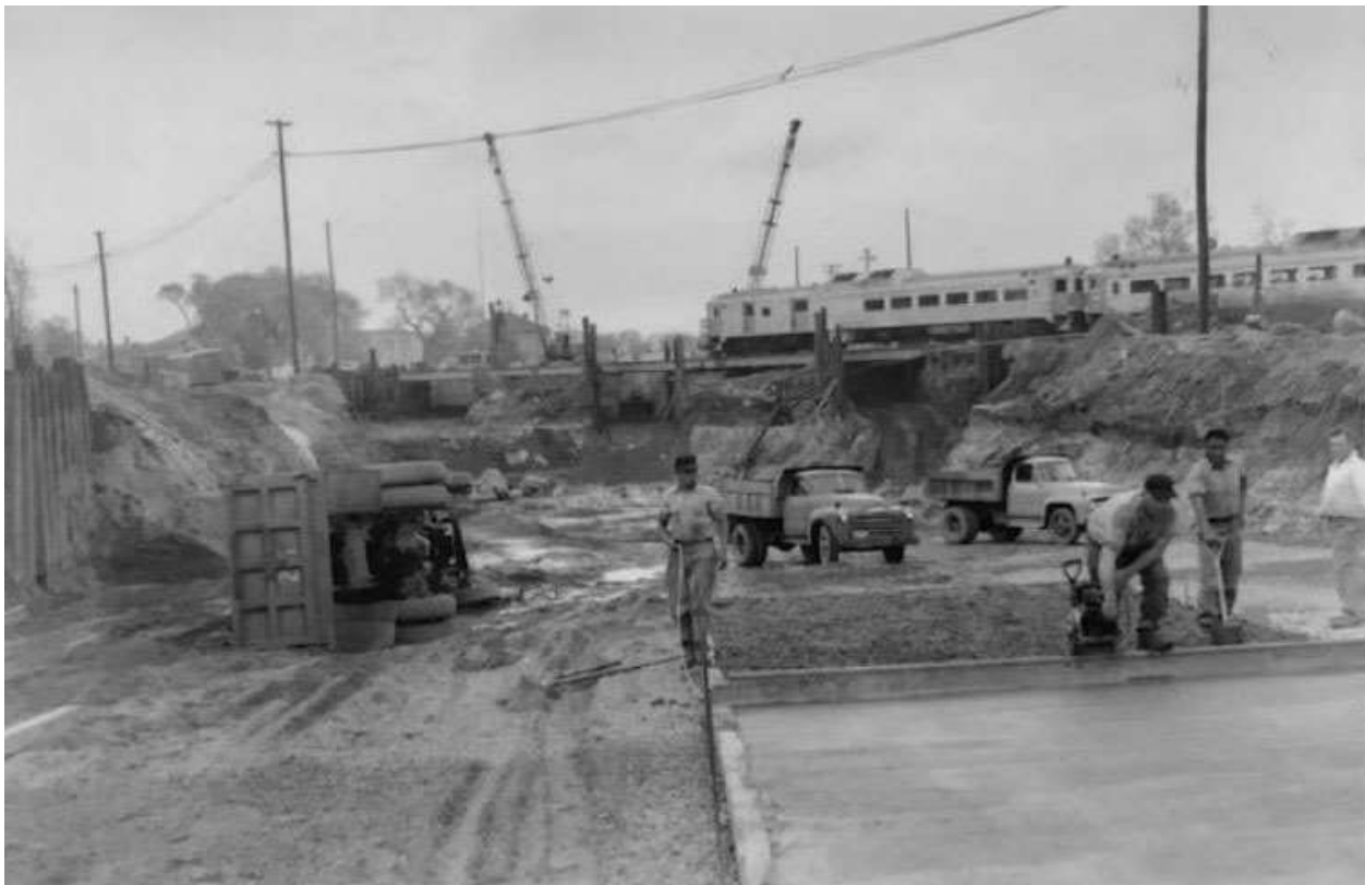
Chauncy Street during construction of the 1950s Underpass project to reduce grade level railroad crossings.
