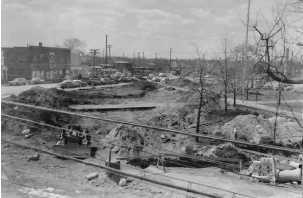
A view of the North Common during the Underpass construction project.
